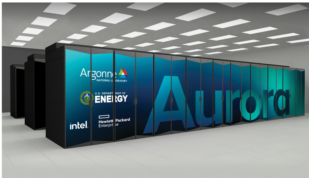
FIGURE 4: Aurora, currently under construction, will be the first exascale computing system in the United States. It will compute a billion billion ( i.e. , a quintillion) operations each second. Credit: Argonne Leadership Computing Facility
